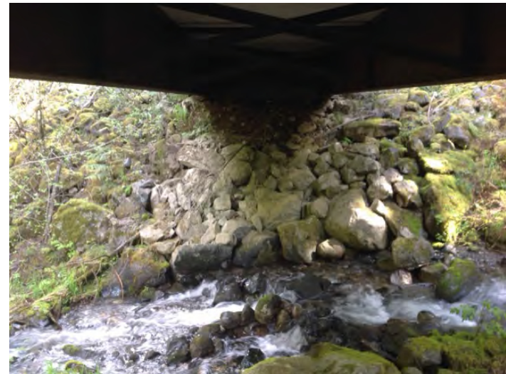
Right Bank Abutment when facing downstream
