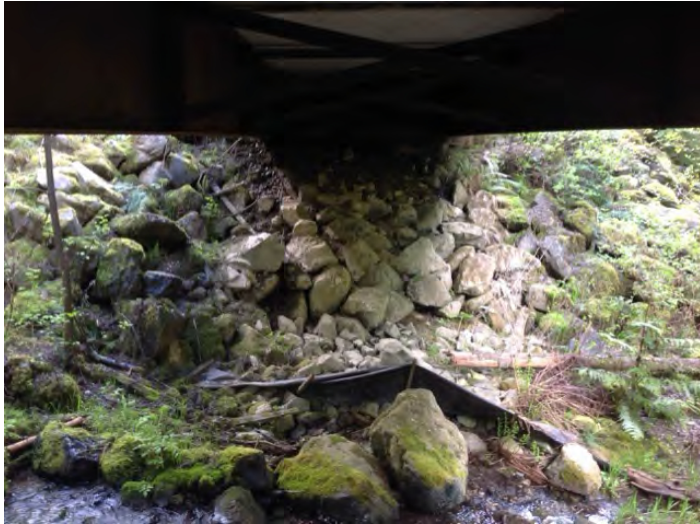
Left Bank Abutment when facing downstream
